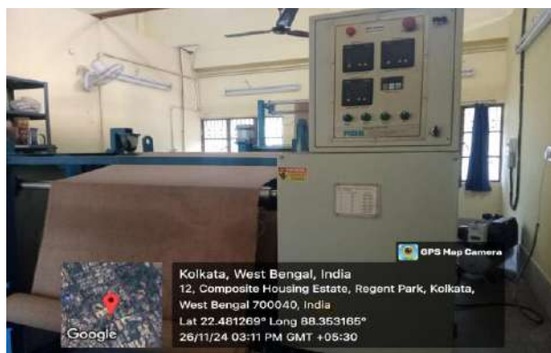
Figure 1b. Drum dryer
